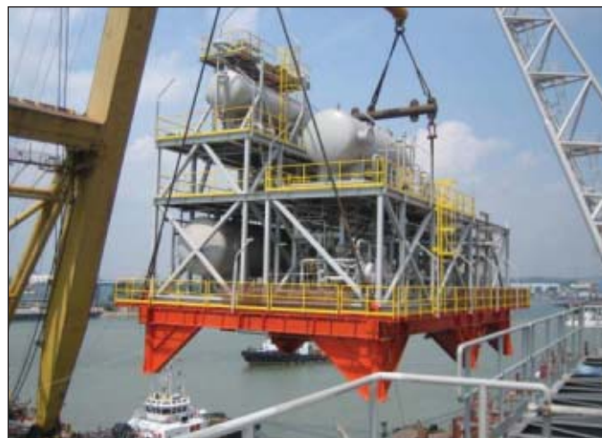
Expro's topsides process module being lifted onto the customer's FPSO. Photo courtesy of Expro.
